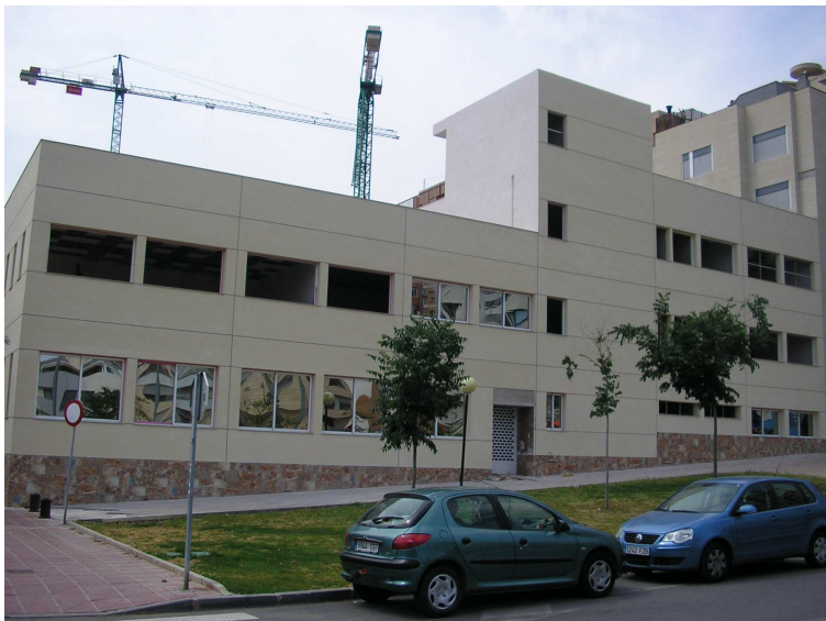
Fachada lateral (mayo 2009)
